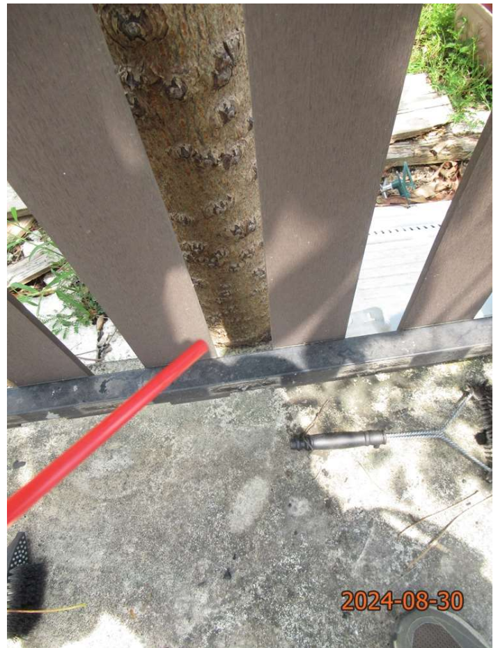
T5 Tree base embedded to concrete structure
